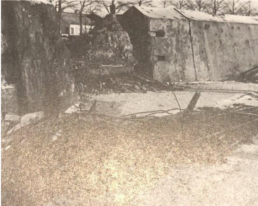
The one bridge left intact over the Zoom, blocked by this concrete barrier.
