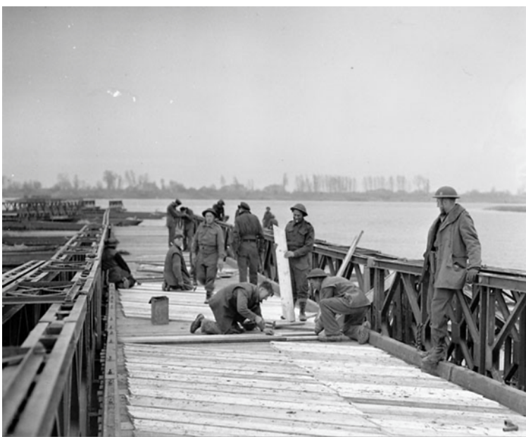
Sappers of the Royal Canadian Engineers lay decking on the Blackfriars Bridge over the Rhine near Rees, Germany. March 30, 1945. © Library and Archives Canada
