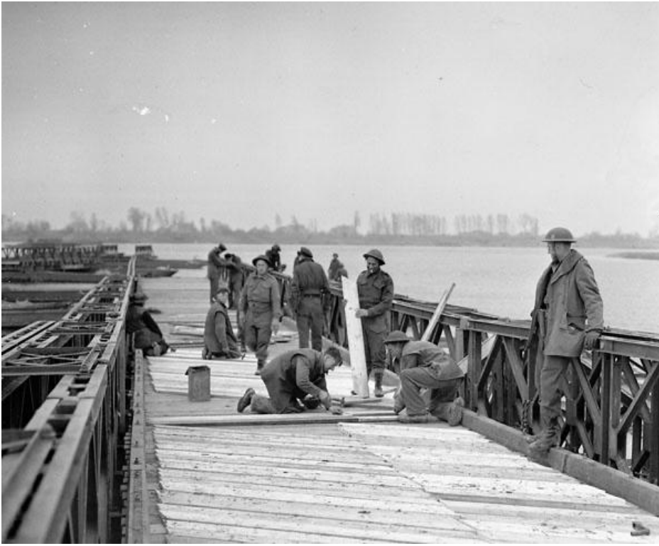
Sappers of the Royal Canadian Engineers lay decking on the Blackfriars Bridge over the Rhine near Rees, Germany. March 30, 1945.
