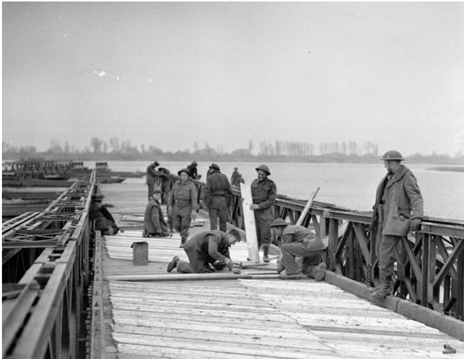
Sappers of the Royal Canadian Engineers lay decking on Blackfriars Bridge over the Rhine at Rees, Germany, om 30 March 1945. Photo Library and Archives Canada
